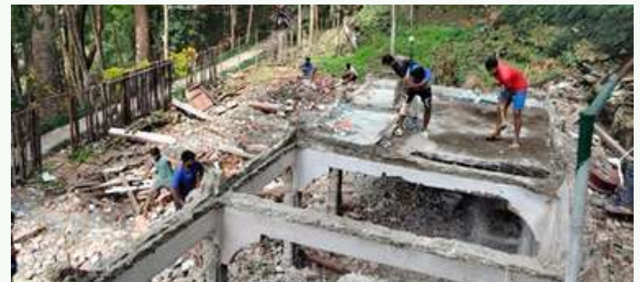
Novices at work- Demolishing the old!
